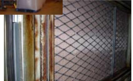
*Contaminant passing through the low efficiency washable filters led the customer to Camfil for a solution to their problems.*
