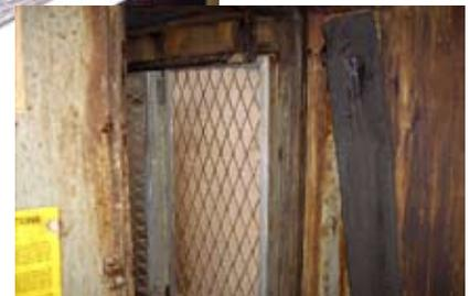
*The caramelization of the byproducts of the manufacturing process created complications for HVAC maintenance and increased the possibility of process compromise due to uncaptured contaminants.*
